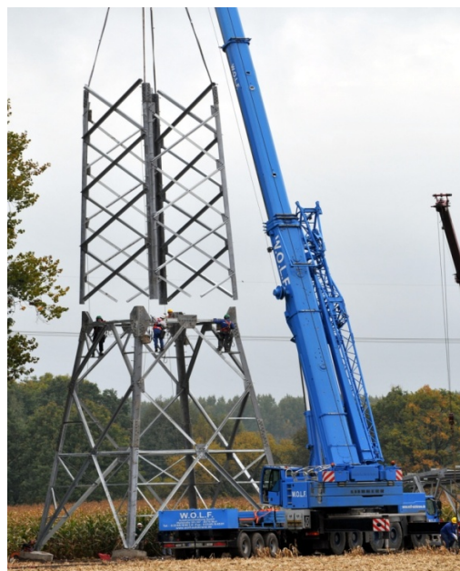
Abb. 7: Mastmontage (Stocken)
